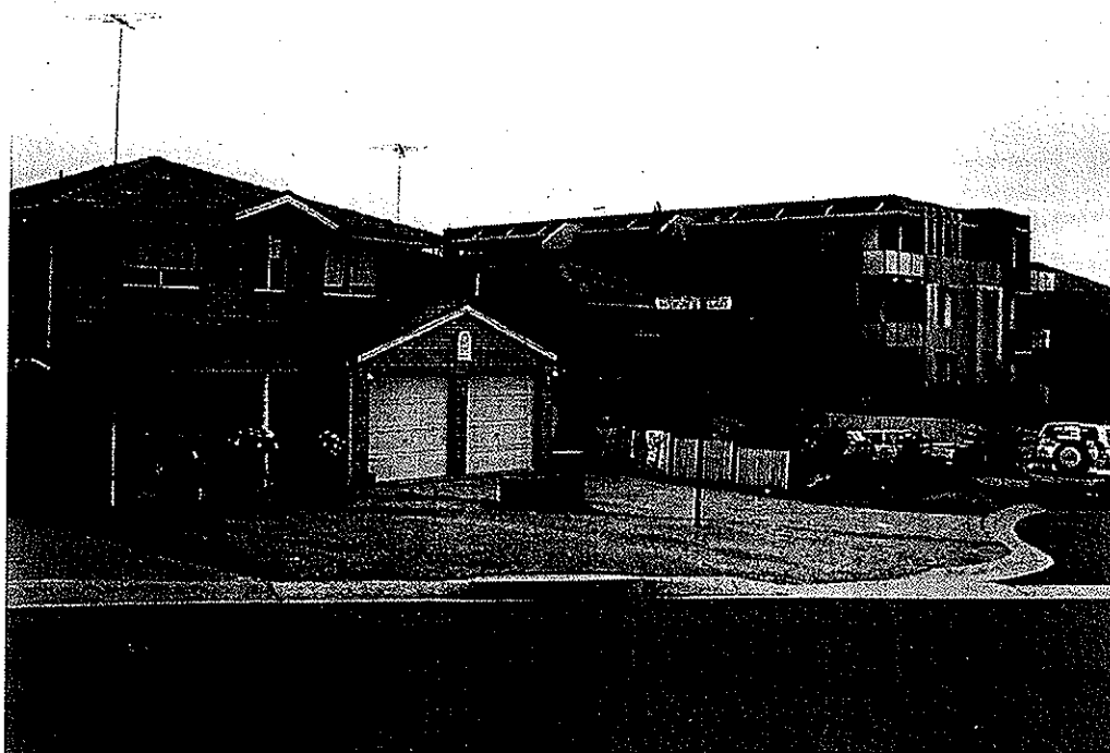
Figure 4 – 1-3 Kilbenny Street and Adjoining RFB
