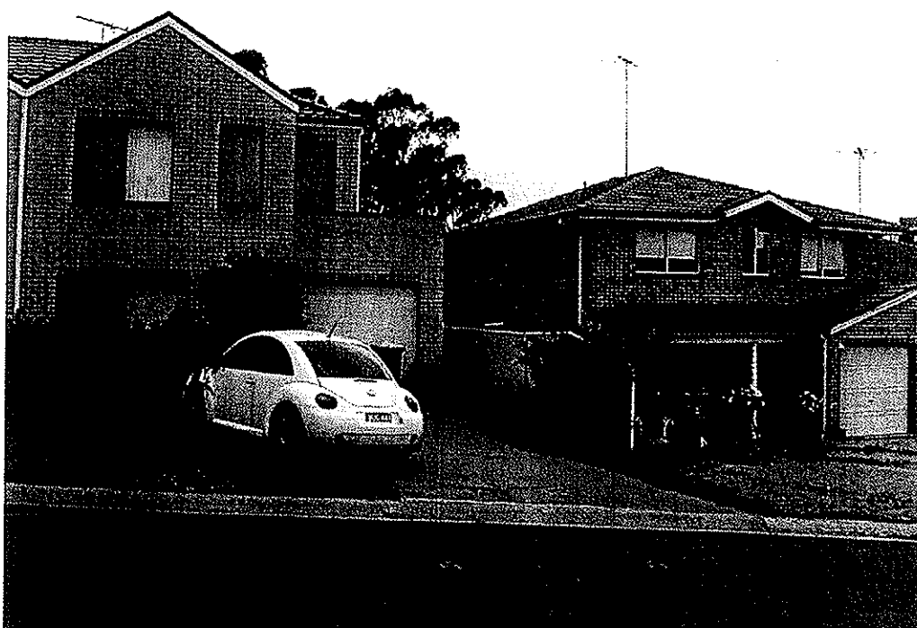
Figure 5 – 1 Kilbenny Street and Adjoining Townhouse Development at 53 Waterford Street
